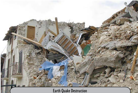
Earth Quake Destruction
