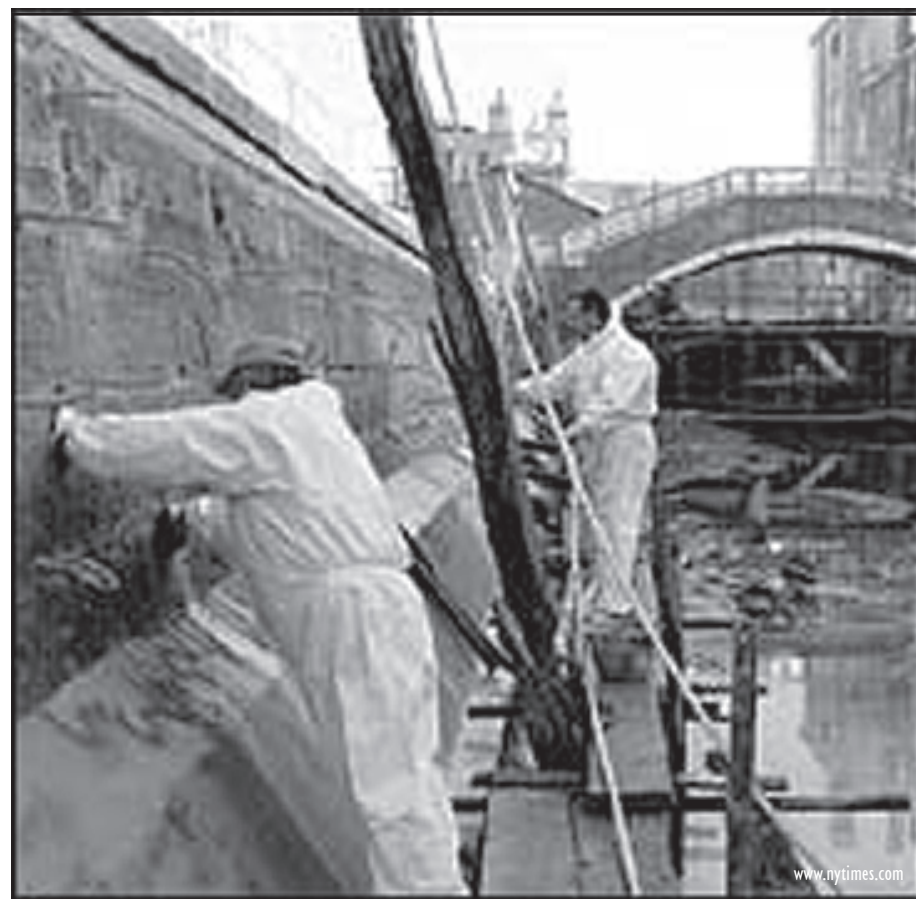
Workers repair the channel of the drained Squero di San Trovaso.
